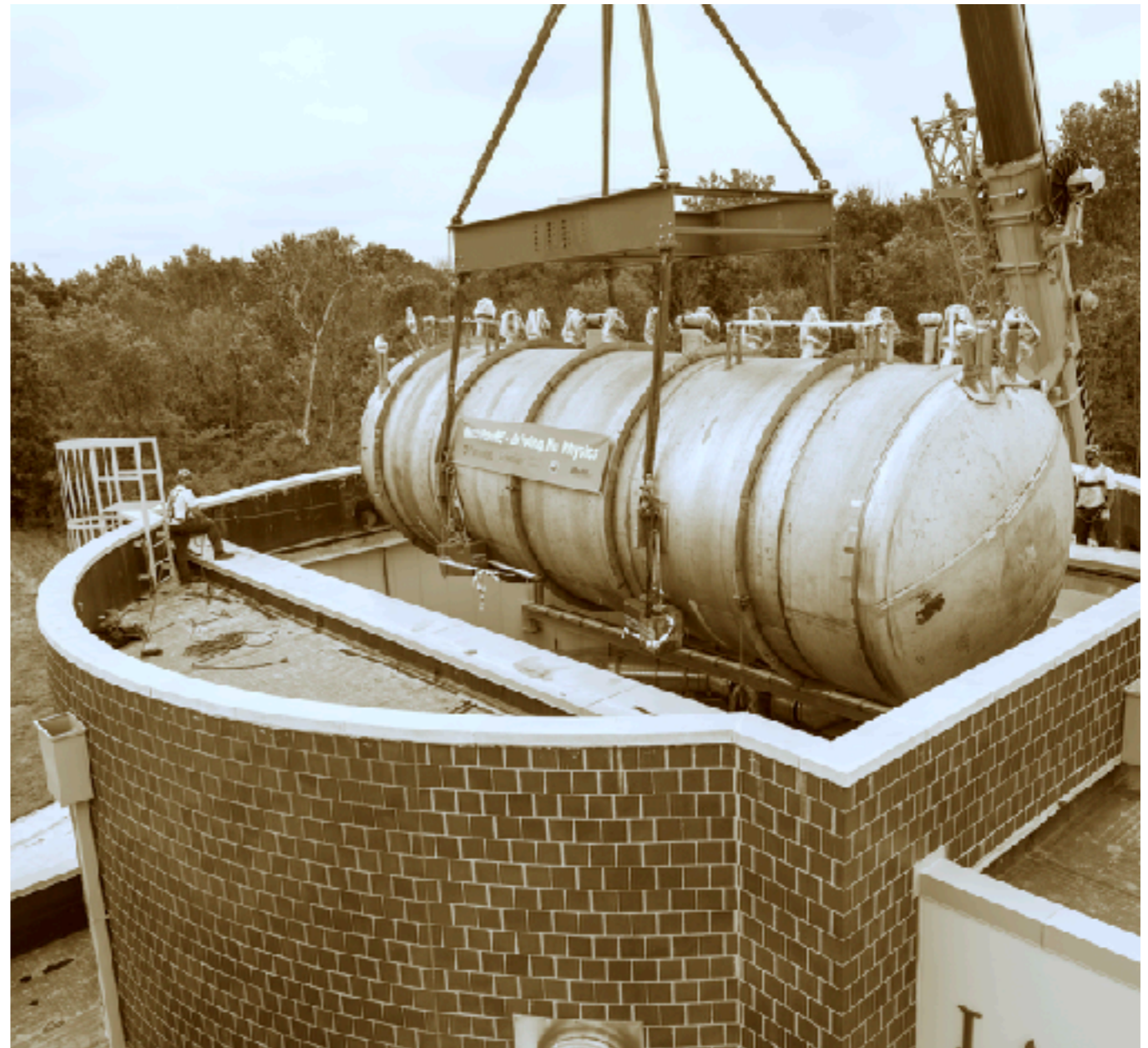
The MicroBooNE cryostat being moved into the Liquid-Argon Test Facility (LArTF).
