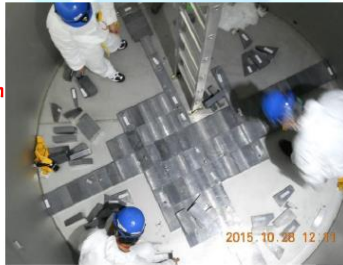
Pb blocks for shielding \gamma -rays
